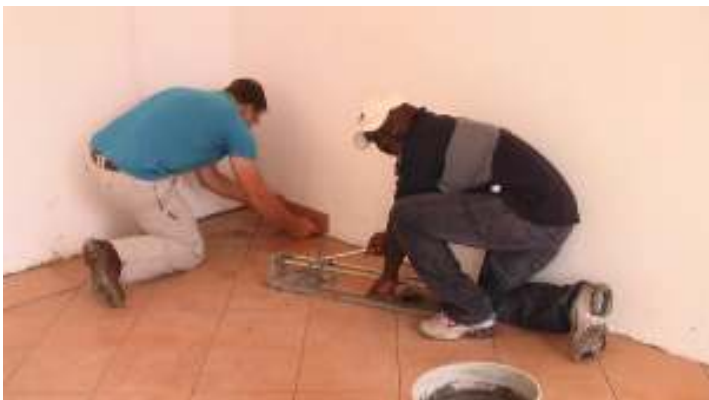
Bro. Kirk and Bro. Jonas laying ceramic tile in new office
