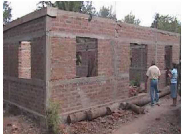
New Church walls complete in Gonja
